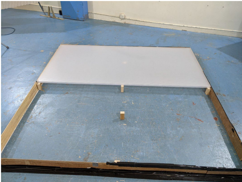
Figure 4 – Specimen partially installed over spacers
